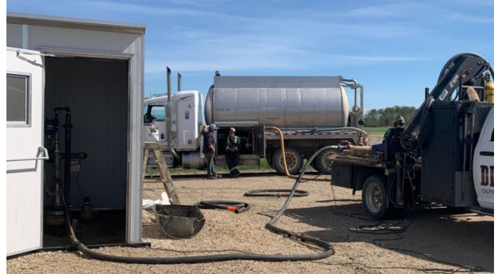
(b) Test setup showing the blowdown tank and H 2 S scrubber
